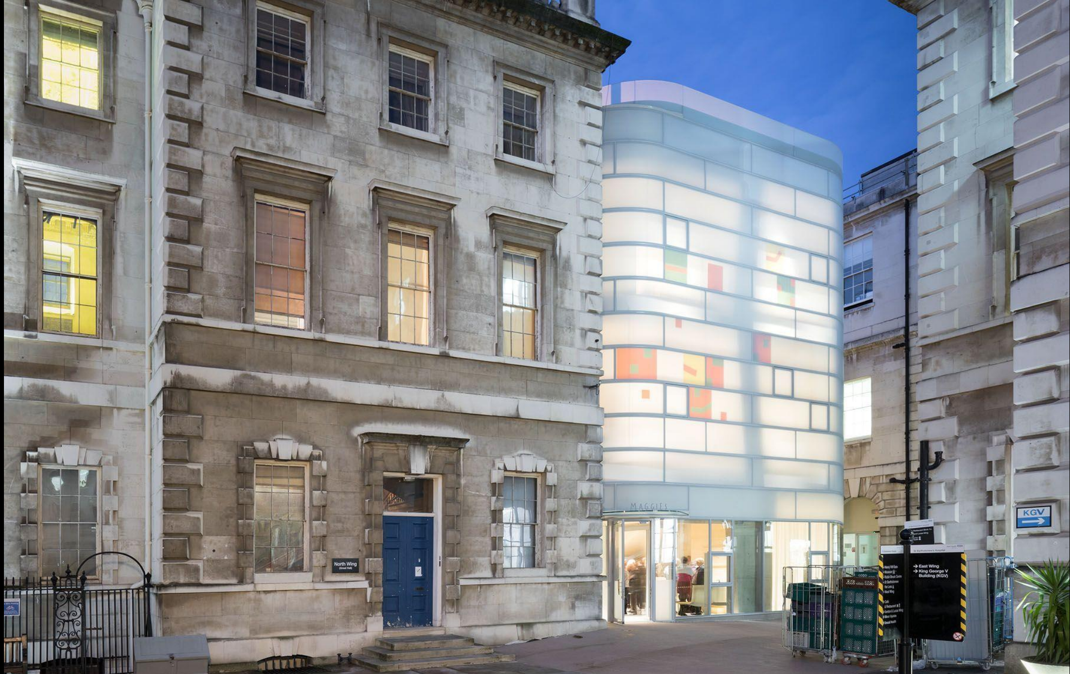
Iwan Baan (Photograph)
